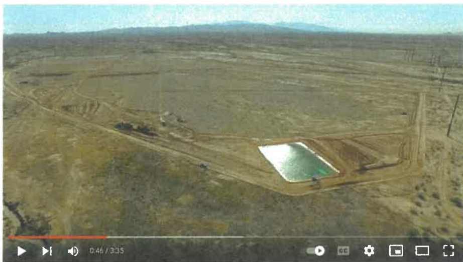
Red Rock Solar Plant Construction Update #1
