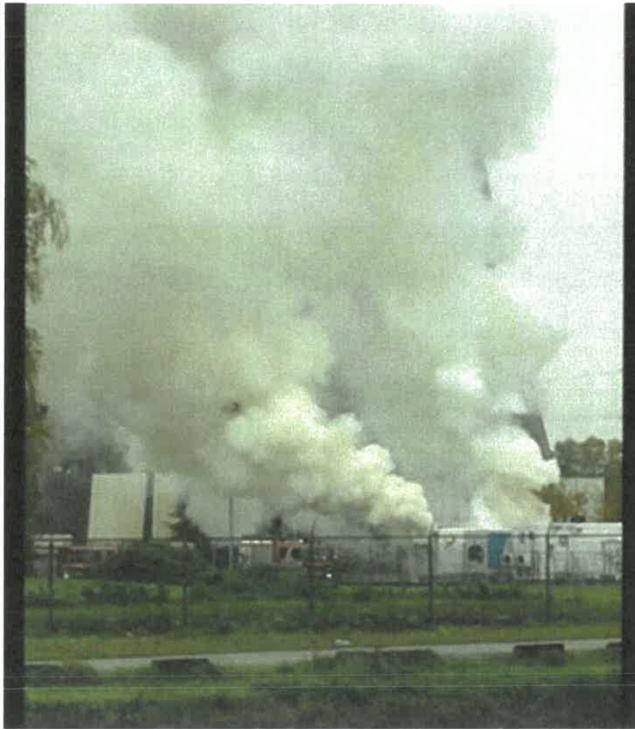
"Battery Fire" at Drogenbos, Belgium 11 Nov 2017. 1 MWh facility; fire occurred during commissioning. Taken at the start of the incident . Image: Wade William Ferguson
